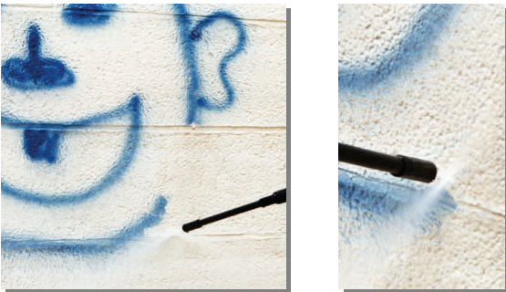
If the protected surface is soiled with graffiti: clean surface with a high pressure cleaner.
