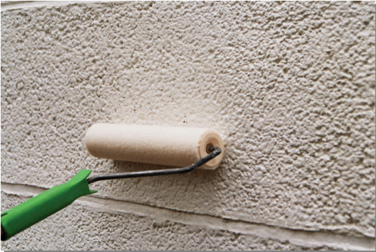
Application of PROWALL , e.g. with a roller.
